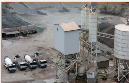
Construction materials industry
