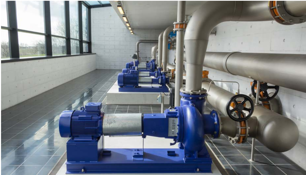
Electrically operated pumps in earthed networks, which are predominantly switched off, cannot be permanently monitored with residual current monitors.
